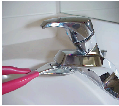
(1) Loosen Filter Screen
