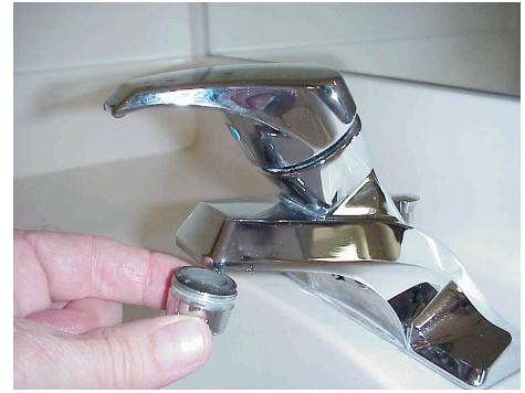
Remove Filter Screen
