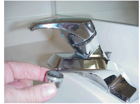
Remove Filter Screen
